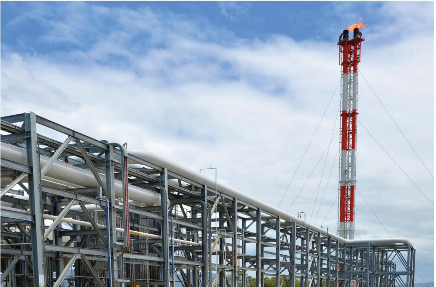
Flaring is an essential part of the LNG production process, ensuring the conversion of natural gas to liquid is carried out safely.
