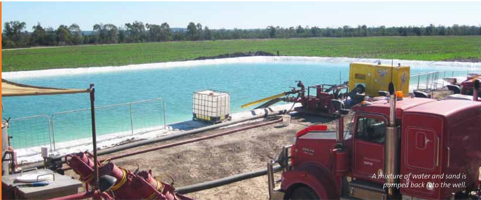
A mixture of water and sand is pumped back into the well.
